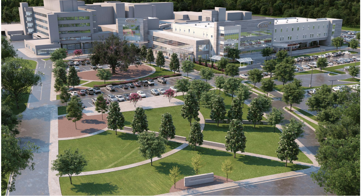
Photo Rendering of SGMC Health's Main Campus expansion, set to be completed in late 2026, courtesy of SGMC Health
